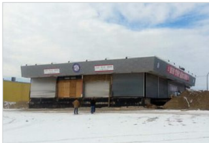
The former arcade location was boarded up after Hurricane Sandy.
