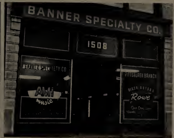
The facade of Banner's Pittsburgh office. Little outside change is evident since the branch was founded in '37 but inside is a different story.
