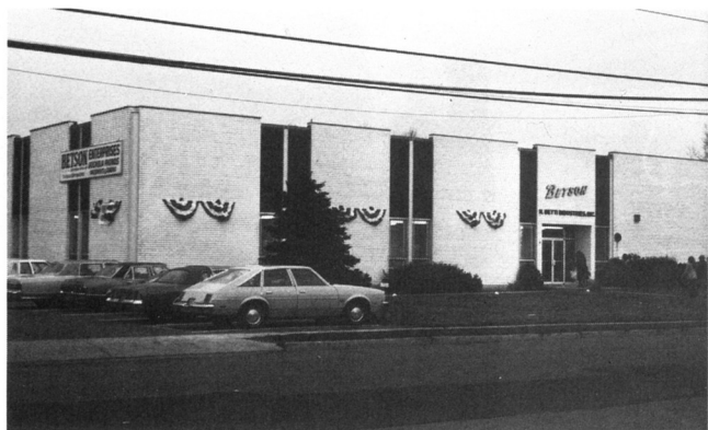
New headquarters for Betson Enterprises features 45,000 square feet of offices, showrooms, and warehouse space.
