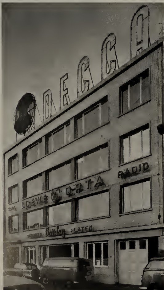
MAIN BUILDING OF S.A. FONIOR IN BRUSSELS
