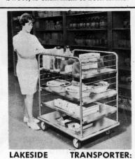
new Lakeside Model 360 Adjustable Shelf Truck, suitable for use as a central supply truck or in a variety foodservice applications, features a top shelf of "4-sidesdown" design, to accommodate shelf dividers; other shelves are "2 long sides up -2 short sides down" style, all fully adjustable in three - inch increments. Another model features underside channel slides for two fiberglass drawers. Trucks are heavy - gauge stainless steel with five-inch swivel casters.
