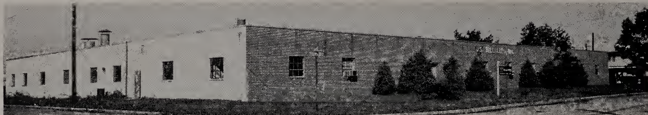
U. S. Billiards' new Amityville plant occupying 50,000 square feet.
