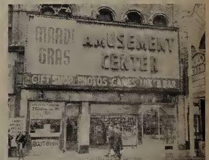
OLD FRONT will come down shortly with new fixtures on order to brighten the appearance.
