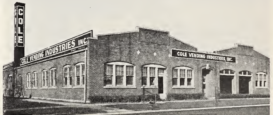
Cole's new plant occupies 14,000 sq. ft. of space.
