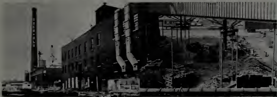
Work progresses on Rock-Ola factory "facelift"
