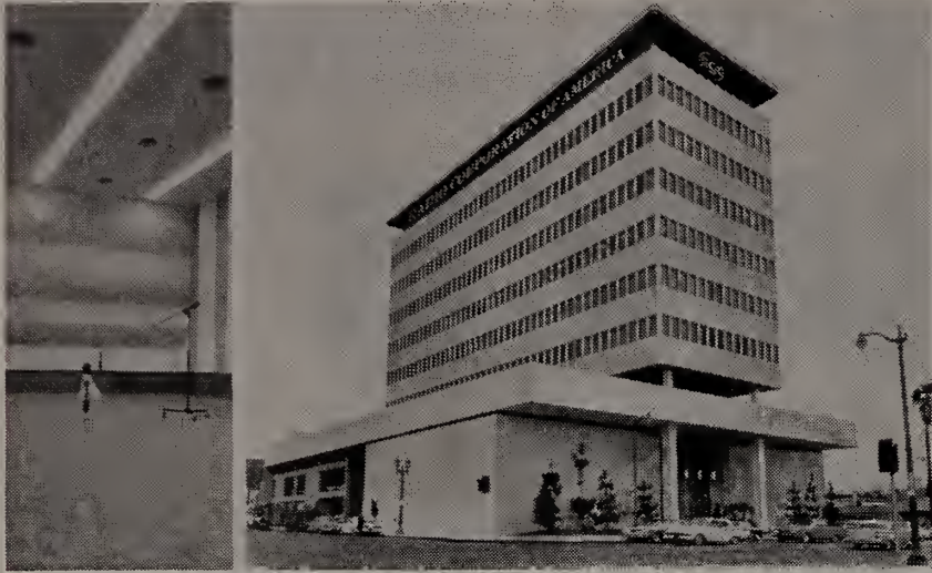
HOLLYWOOD—RCA Victor's spanking new headquarters in Hollywood (6363 Sunset Blvd) is ready for business. Photos show a view of the smart-looking edifice and the large studio space, which is emphasized by the appearance there of Vera Kilpatrick, Victor's new, 5-year-old singing tot.
