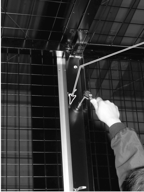
PHOTO 6-7b 2 bolts at upper side
