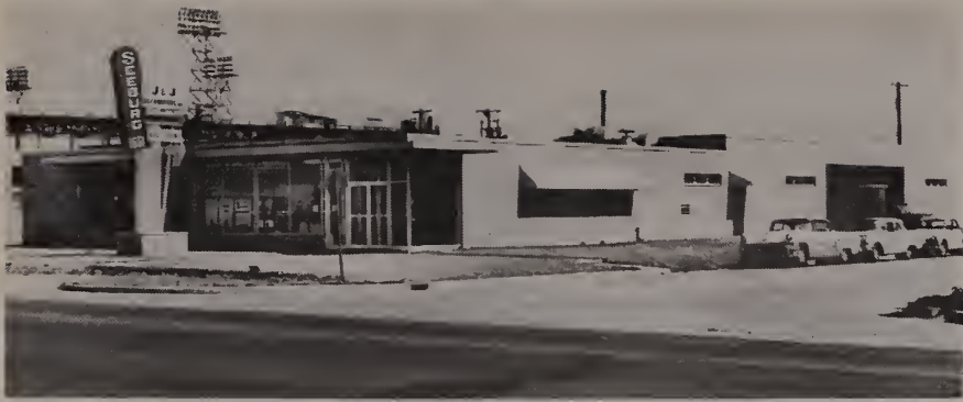
The new home of J & J Distributors, Inc. is a modern one-story brick building with 14,500 sq. ft. of floor space.
