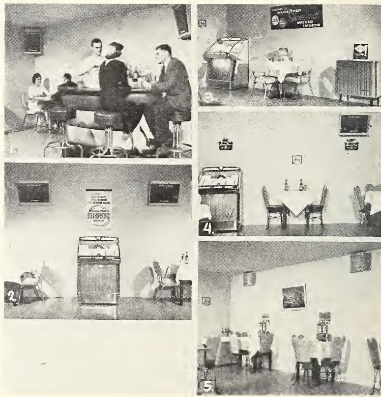
Pictured above are five different type installations. #1—Indicates a typical small room separated from the phonograph itself. Here, two model "5124" Corner Speakers serves as Channels A & B to give complete stereophonic music coverage throughout the room. #2—Shows a 200-selection stereo phonograph muted with two model "5123" Wall Speakers carrying Channels A & B. Such an installation often uses extender speakers to complete the stereo system. #3—This very simple stereo installation shows a model "2300S" phonograph used in conjunction with a Console Floor Speaker model "5122". Both units face directly down the room. #4—Demonstrates an installation using a phonograph as Channel A and a "5123" Wall Speaker as Channel B. #5—Shows extender speakers model "5125", which are placed so as to reinforce the music in other parts of the location. This installation also includes model "5252", 200-selection dual pricing wall boxes with wall cards calling attention to the new Stereo Music System.
