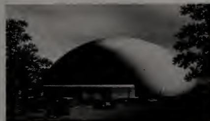
A LOOK AT TOMORROW — Houston, Texas will soon offer the world's largest motion picture sound stage, shown here in an artists' rendition. Designed by Aeschbacher Chambers Architects and built by Temcor, the domed facility is scheduled for completion in early 1986.
