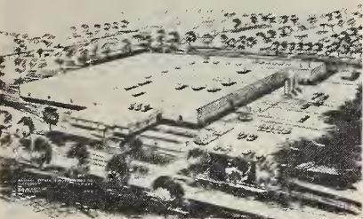
Mercury's new Richmond plant.
