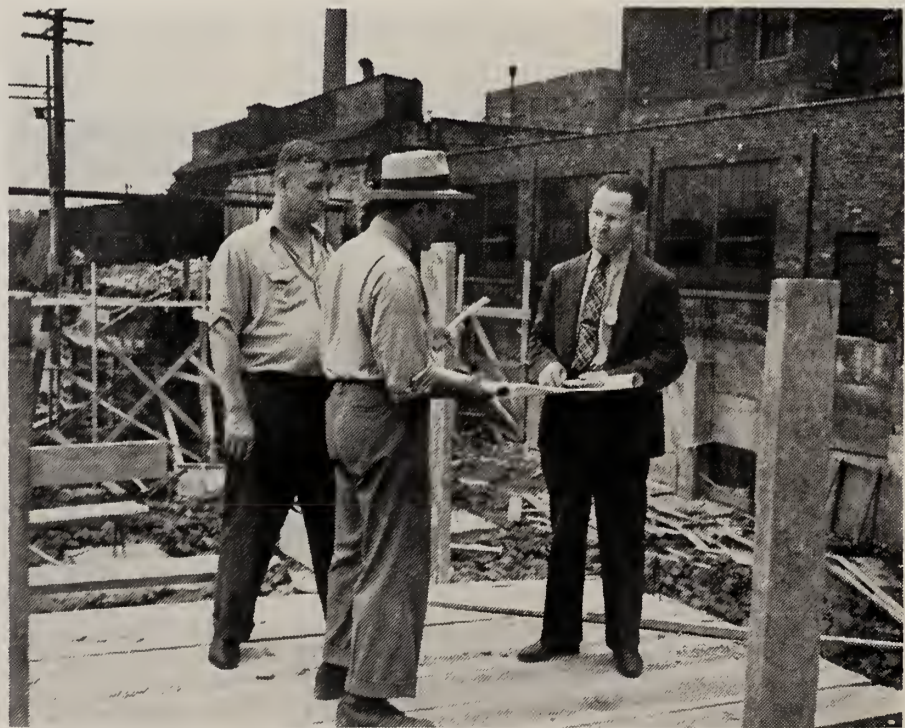
In 1942 expansion plans were underway at the Rock-Ola factory (above) paving the way for future growth which eventually led to the present size plant (upper right opposite page) which today occupies several square blocks of area within the City of Chicago.
