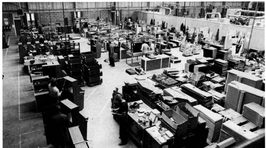
The cabinet shop inside Bell-Fruit's new facility in Nottingham
