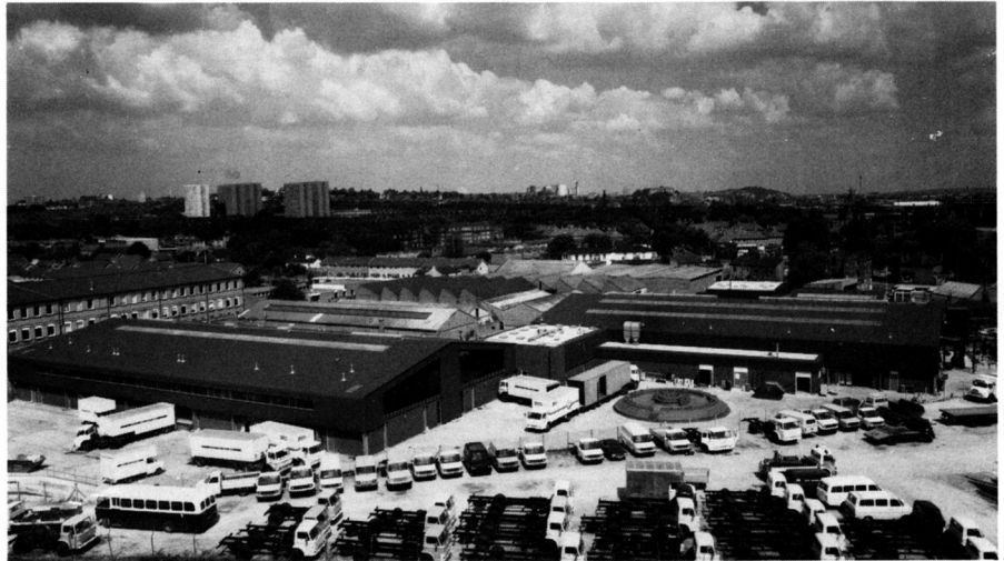
An outside view of the new 60,000-square-foot extension of Bell-Fruit's Nottingham factory
