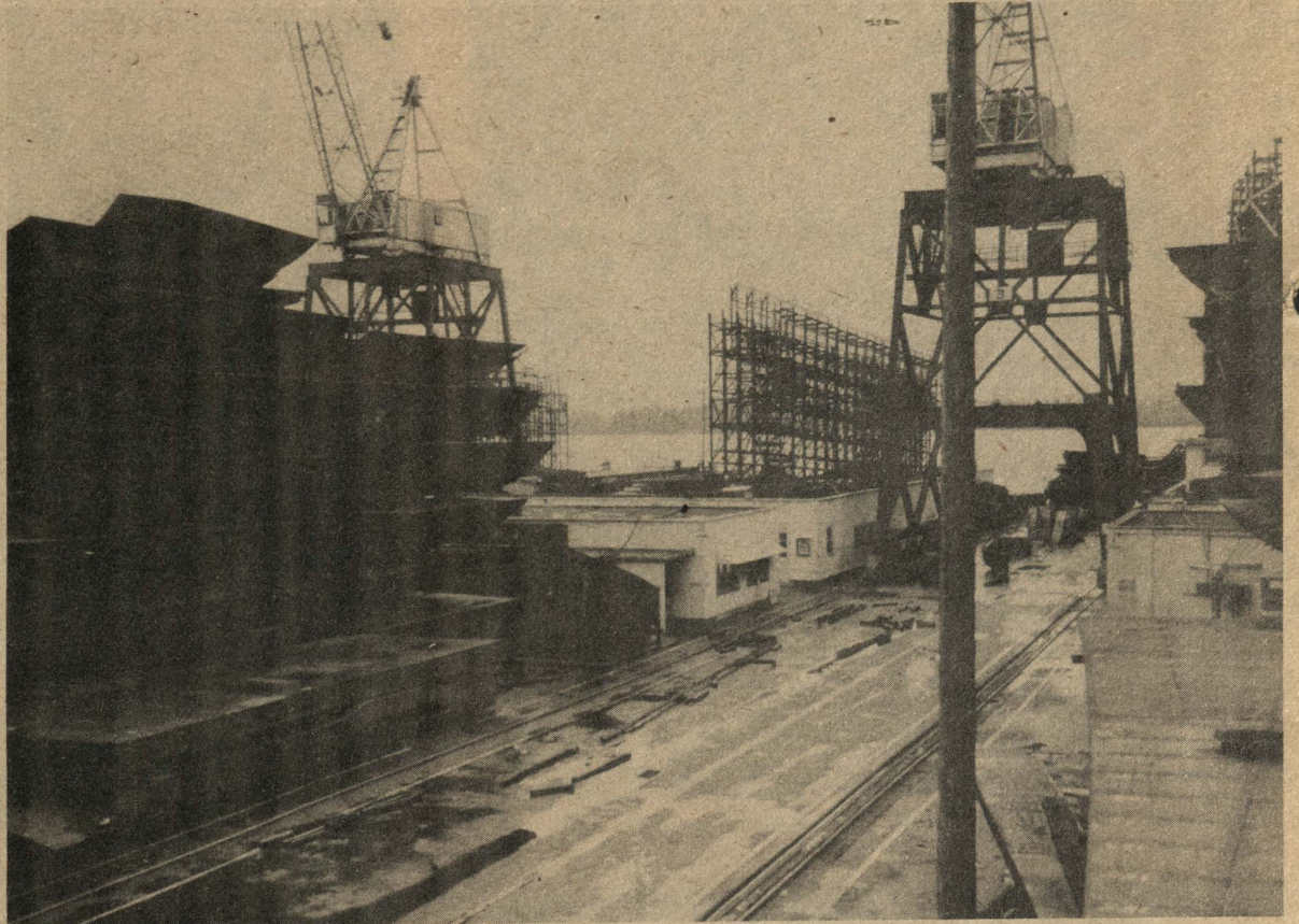
Everything Must End — Tons of steel, fabricated for vessels that might have carried American boys to bloody shores of Japan had not the A-bomb ended the war, stand as stark testimony in front of Ways 3 and 4, now dismantled except for the one small arm of the "Christmas tree" scaffolding visible in the background. The sections in the foreground are keel plates and tank top for originally scheduled C-4 vessels.
