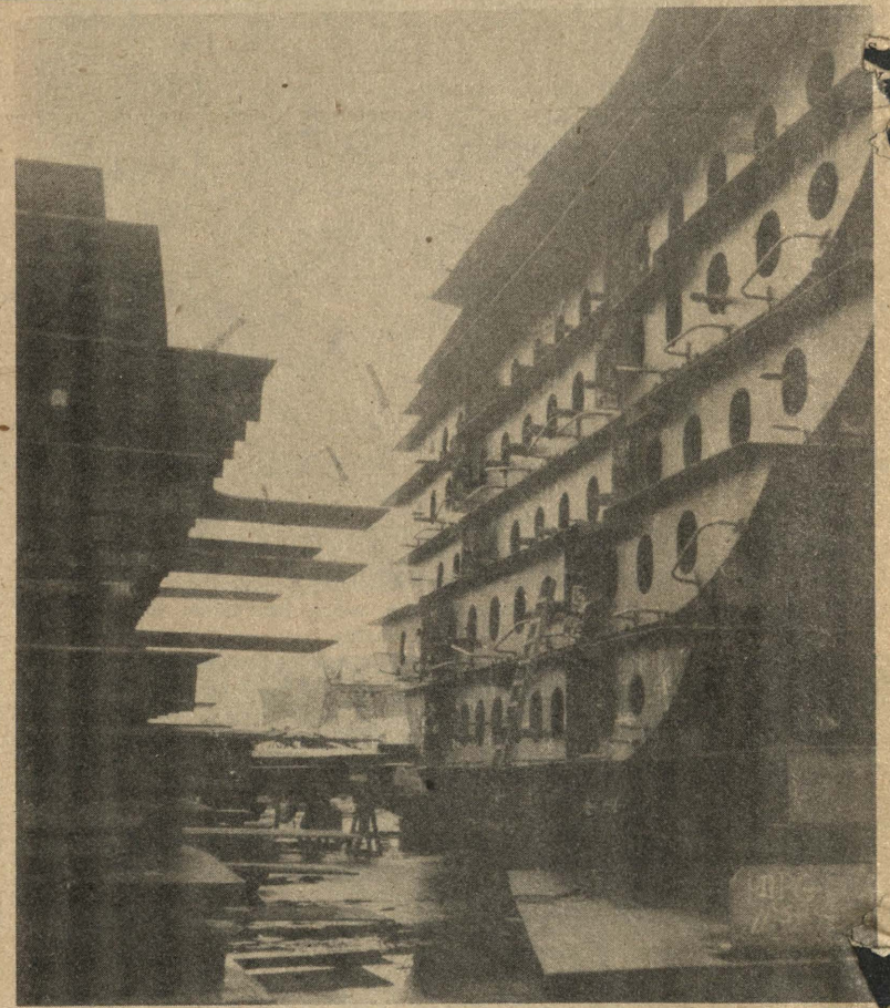
Ways Near End — Vancouver's last two C-4s are barely visible between the piles of never-to-be-used inner bottoms and keel plates for a cancelled vessel originally slated for Way 4. The last of the two C-4s showing in this picture will slide tomorrow (Saturday) at 6 p.m.
