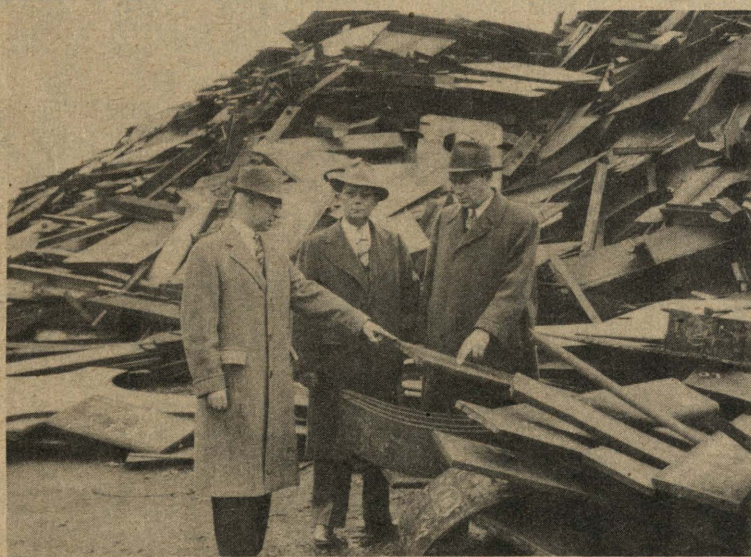
Louis Dulien, Seattle, here points a finger at a piece of steel in the 35,000 ton heap at Oregon Ship for which he bid $8.17 a long ton. Others pictured are Irving Kulp, Dulien's Portland manager, and (right) A. C. McVean, OSC material controller.
