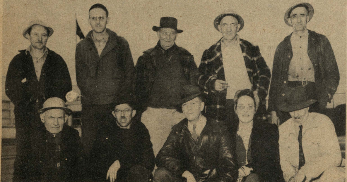
Boiler Men Say Goodbye Here are all the last members of Oregon Ship's Boiler Erection crew, which built 910 boilers weighing 32,270 tons for 455 OSC vessels. Front row, from left, D. H. Ledford, K. M. Vincent, Frank Cour, department superintendent, Gladys Bjornstad, clerk, and Tom Caton. Rear, Herb Miller, Charles Remington; Foreman Roy Wilehart and Thomas Croke. Absent was Wm. Laughter.
