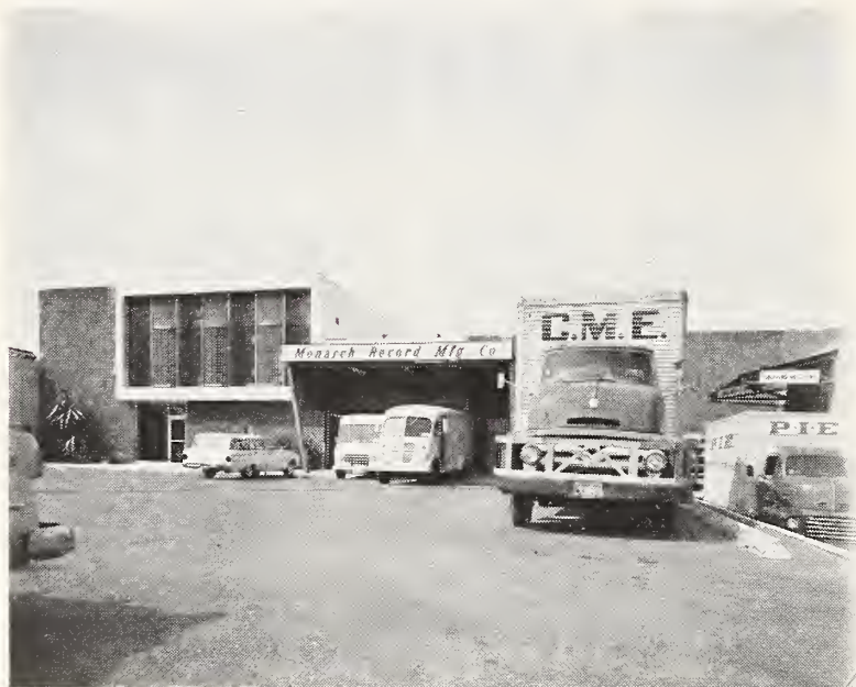
1. View of one of Monarch's buildings, showing loading area and entrance to offices.
