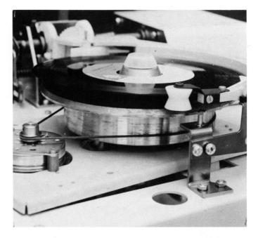
ONE OF THE LATEST improvements in the new German Wurlitzers has been the simplified record changer mechanism, which improves the machine's reliability by utilizing a synchronous turntable motor as used in high-performance hi-fi installations, according to Deutsche Wurlitzer.
