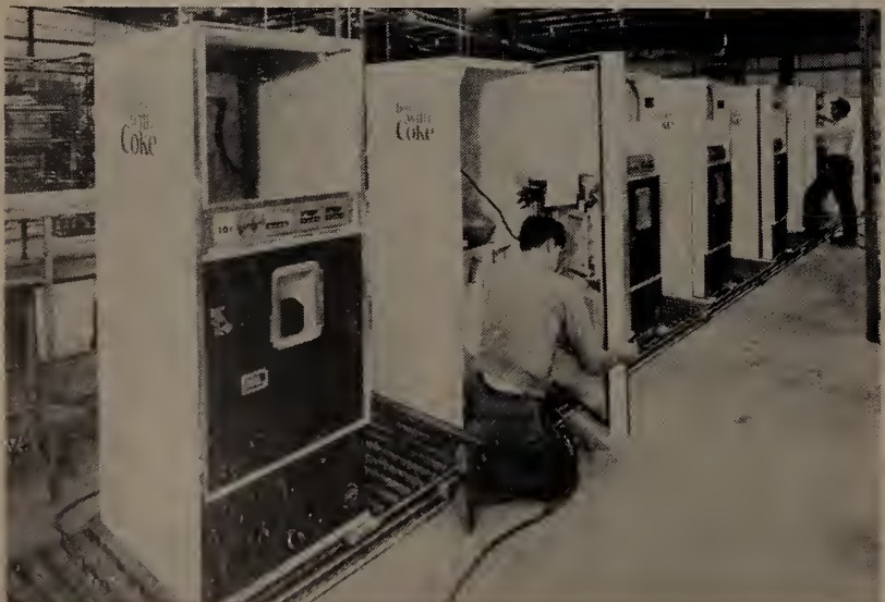
Left: A mechanic gives a careful last minute check on a row of StyleStar Cola vendors before they are packaged for delivery. Down at the other end a second mechanic works. When both meet, the line is certified OK. Right: Packaged and padded, the vendors await loading for shipping out to customers and locations.
