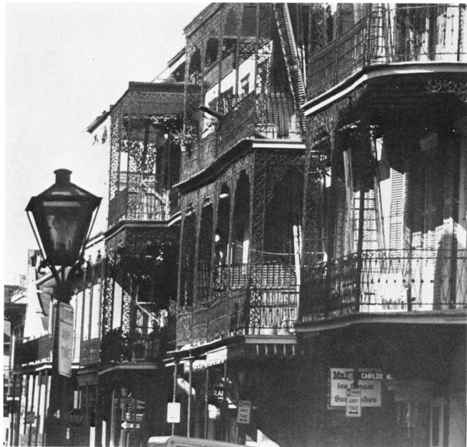
Iron grillework is a noted architectural feature typical of New Orleans: evidenced here on a French Quarter street.
